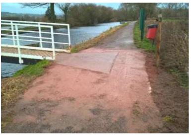
Lift Bridge was resurfaced to bring it up to the same level as the concrete pad, which had begun to stand proud and create a trip hazard.
